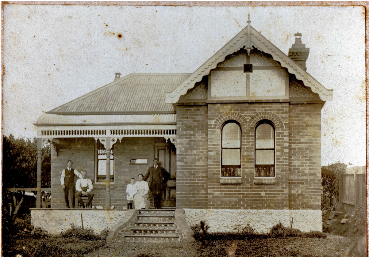
9 Highgate Street, Bexley (c. 1916)
